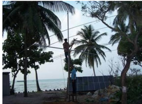
*Installation of 7 element yagi at Panchayat Shack, Minicoy*
